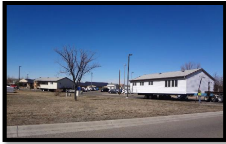
Housing units being prepared for transportation in Montana.
